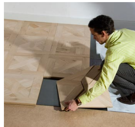
'Elastilon Basic' is used to install regular, solid hardwood flooring, even in the form of artistic parquet squares.
