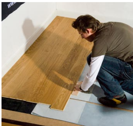
Wooden flooring on Elastilon can be fixed either by removing the protective layer after two rows have been locked together or by just stepping on the surface of the installed parquet.
