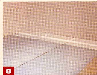
8 Position the auxiliary film.
