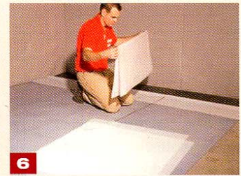
6 Fold the auxiliary film in two.
