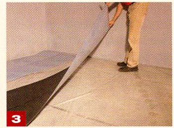
3 Turn over the Elastilon so that the smooth protective layer is on the upper side.
