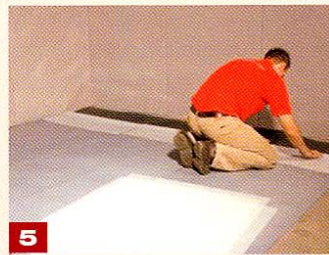
5 Fold back the protective foil of the adhesive layer over a width of one or two boards. The adhesive layer is now exposed.
