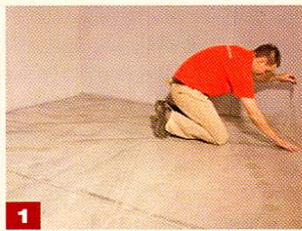
1 Place the polyethylene film on the sub-floor in strips with an overlap of 20 to 25 cm.
