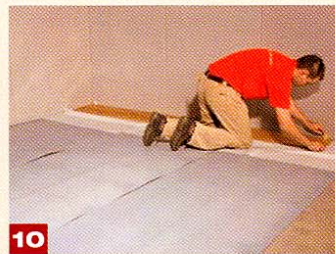
10 Place spacers between the wall and the parquet flooring.
