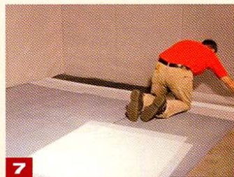
7 Carefully place the auxiliary film onto the exposed adhesive layer with the fold facing the wall
